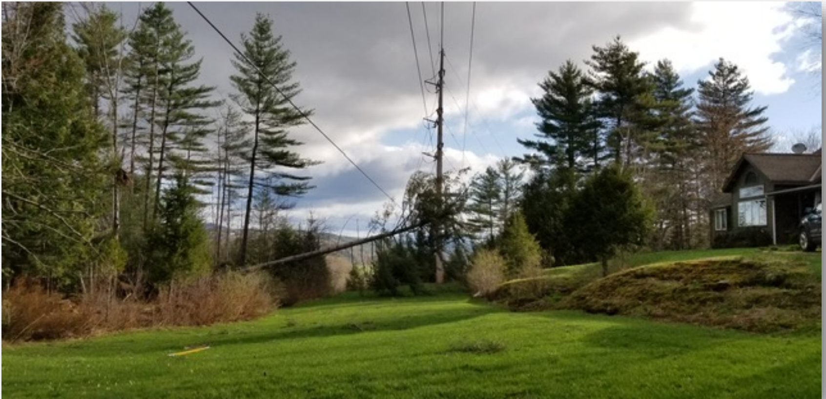
Tree contact on the K24 (Duxbury to Stowe)
