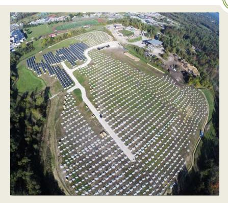
Concrete ballast mount to avoid penetrating landfill cap
